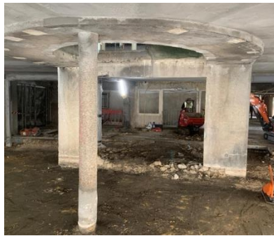
Reinstating the ground to first floor Spiral Staircase, removed in the 1960's
