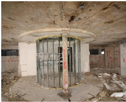
Reinstating the ground to first floor Spiral Staircase, removed in the 1960's
