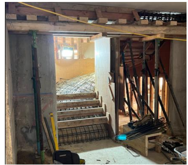
Reinstating the ground to first floor Spiral Staircase, removed in the 1960's
